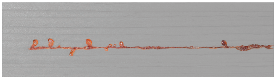
Fig. 2 Pitch or resin on painted surfaces can be easily removed using a clean rag and mineral spirits or turpentine.
